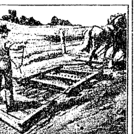
The Spiked Forward Part of the Drag Loosens the Road Soil, and the Following Rear Portion Packs it to a Smooth Surface, Thus Finishing the Surface in One Operation.
